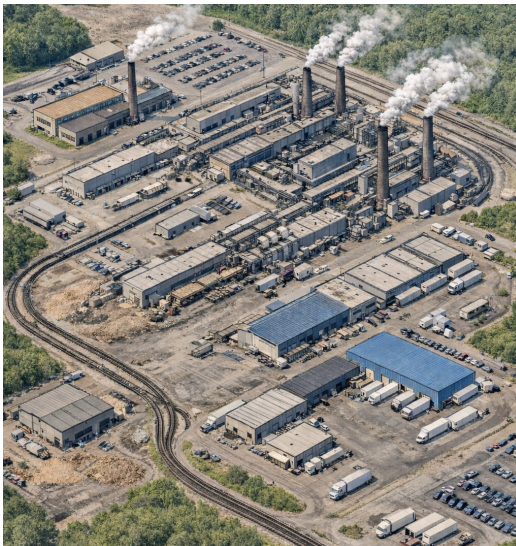
Drone photograph of Rodgers Paper Mill
